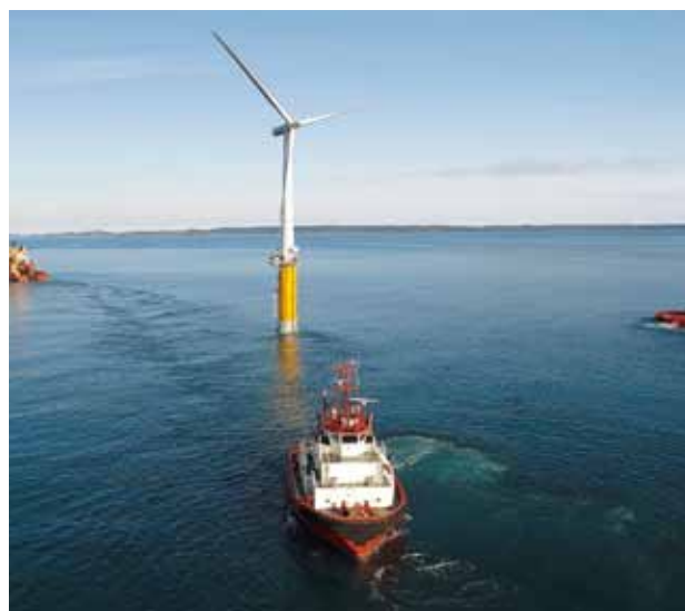
tured and supplied an innovative high-tech wind turbine for a pilot project off the coast of Norway. Anchored in 220 meters of water, the floating turbine is heralding a new era in wind power (see also page 28 of Book I).
