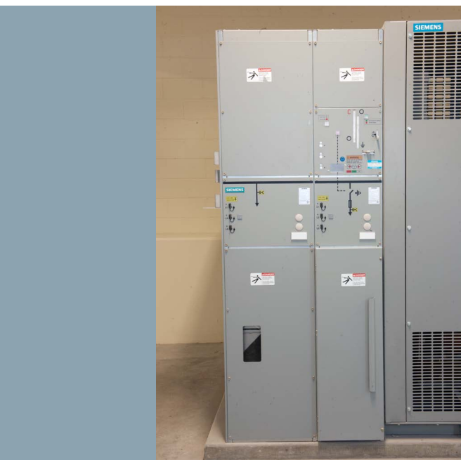
Type SIMOSEC medium-voltage, load-interrupter switchgear indoor installation on raised housekeeping pad.
