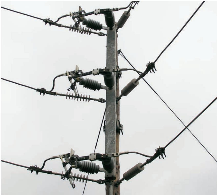
Figure 1: Typical type Vector manual group-operated switch
