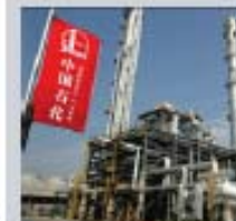
Sinopec Refinery Qsingtiao China
