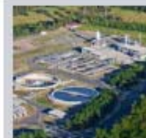
Gold Coast City Council Water- treatment Australia
